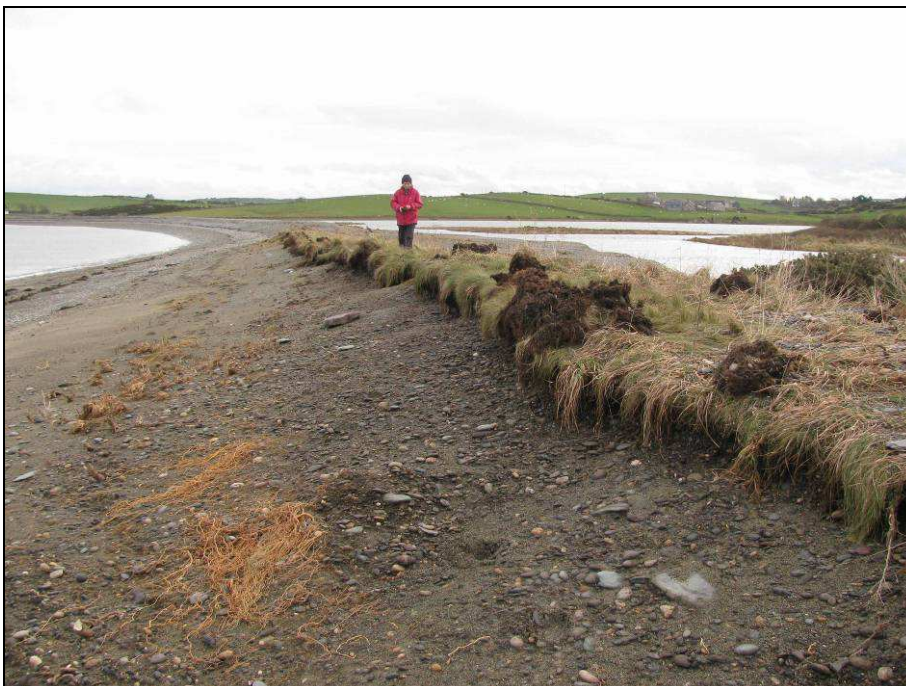
Figure 25. Vegetated shingle ridge at Cemlyn showing erosion at the west end (Ivor Rees, 7 th Dec 2013).
