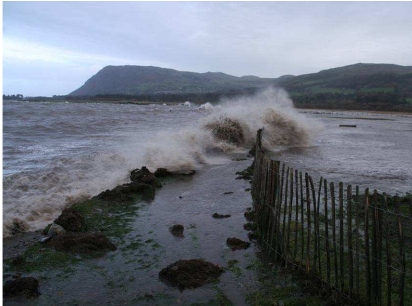
Figure 20. Overtopping of the floodbanks at Morfa Madryn, Llanfairfechan (John Ratcliffe, Natural Resources Wales. 5 th Dec 2013).
