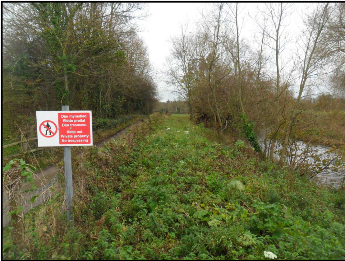
Plate 3.16: Existing embankment near Dol Afon footbridge
