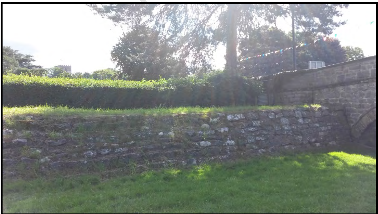
Plate 3.11: Stone pitching to be removed and reinstated
