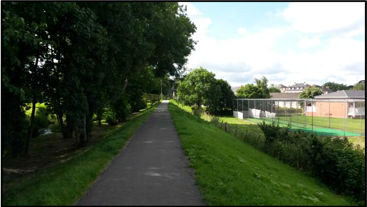
Plate 3.6: Existing embankment and footpath facing south towards Pont Begard footbridge
