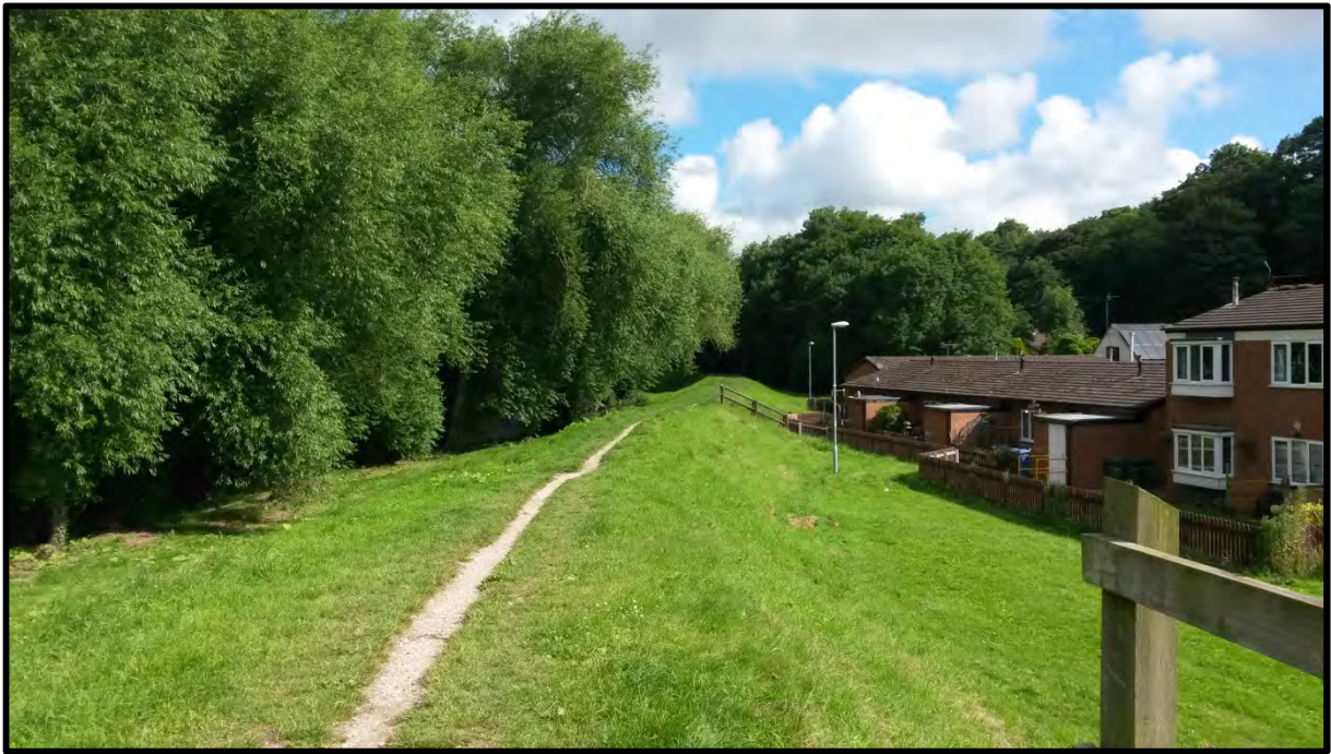
Plate 3.13: Embankment behind properties at Mill Street, facing north
