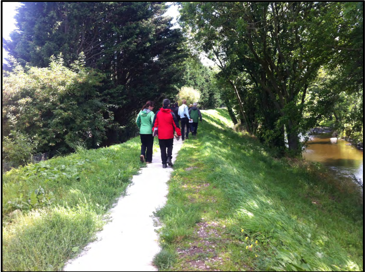
Plate 3.14: Existing embankment behind Dwr Cymru Welsh Water Sewage Treatment Works
