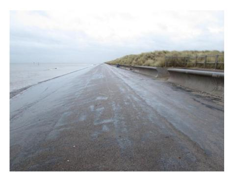
Figure 26. Gently sloping revetment and low wave return wall at Frith Beach, Prestatyn, which allows blown sand from the beach to reach the dunes
