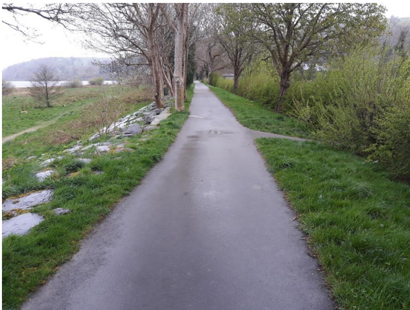
Plate 2.3: Lake embankment, looking west
