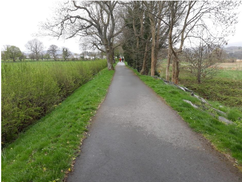
Plate 2.2: Lake embankment, looking east
