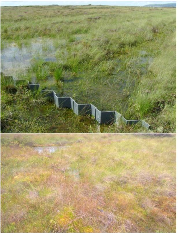
Figure 7. Above – Cutting one year after piling installed. Below – Cutting ten years after pilling installed.
